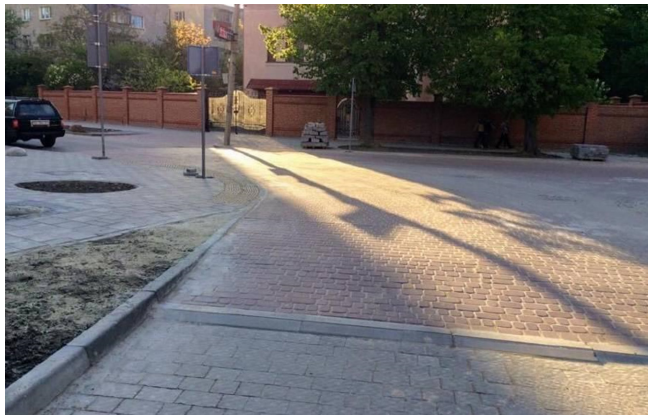
Fig. 6.16 Crossroads with a raised roadway level [26]
